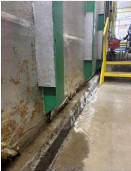
Photos of the steel water treatment plant tanks showing the pitting, corrosion, and leaks in the tanks
