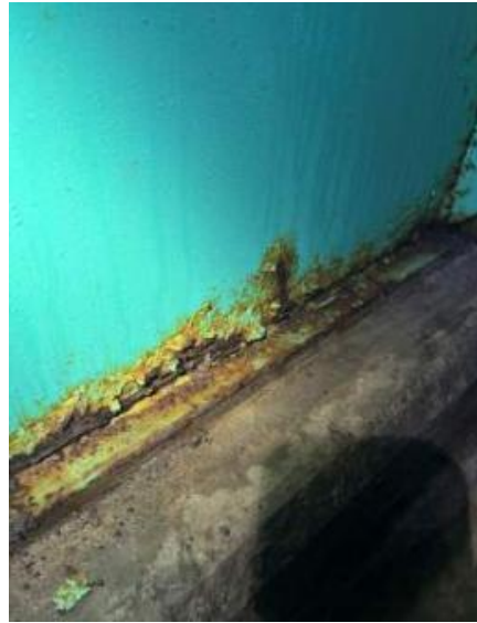
Photos of the steel water treatment plant tanks showing the pitting, corrosion, and leaks in the tanks
