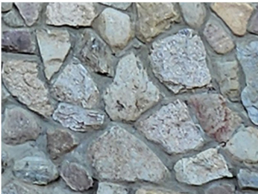
Existing Stone Veneer Base
